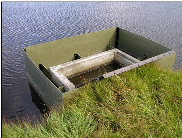
Photo 1: Overflow Structure at Regional Stormwater Pond
